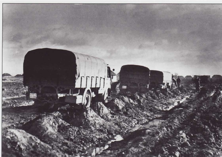
Cargo trucks haul supplies to the front. The mounds alongside the road are spoil from digging a drainage ditch for the spring flooding. The gaps between the mounds allow for drainage from the road's surface.
