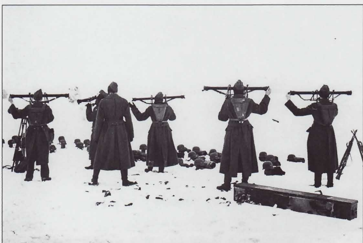
A field training school for 2cm or 3.7cm Flak gun aimers. They are training with the 1-meter Em.R. stereoscopic rangefinder. The triangular tan or brown leather cases on their backs are for the folding shoulder rests. The rangefinder itself would be slung over the shoulder by a carrying sling.
