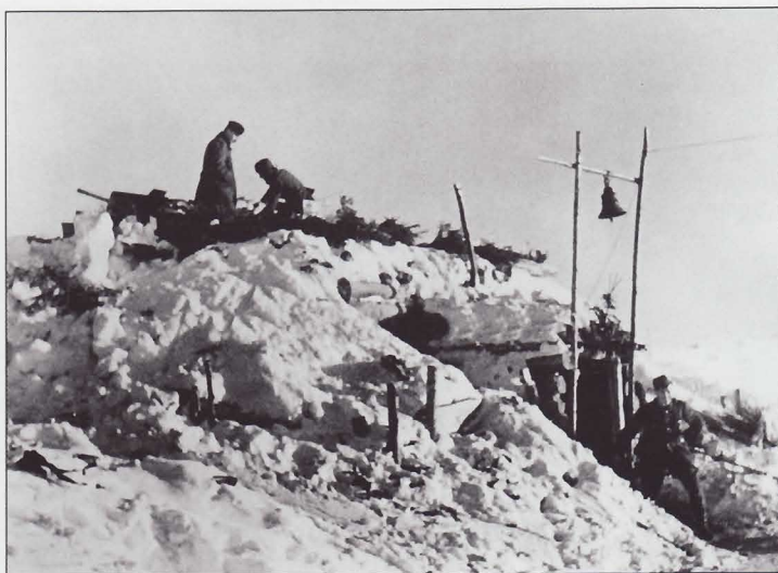
This 2cm Flak 30 position was built atop a bunker of heavy timbers and banked by snow. A bell taken from a church serves as an air raid warning bell. It would take a direct medium caliber artillery shell to knock out such a bunker. The thick covering of snow provided a great deal of protection.
