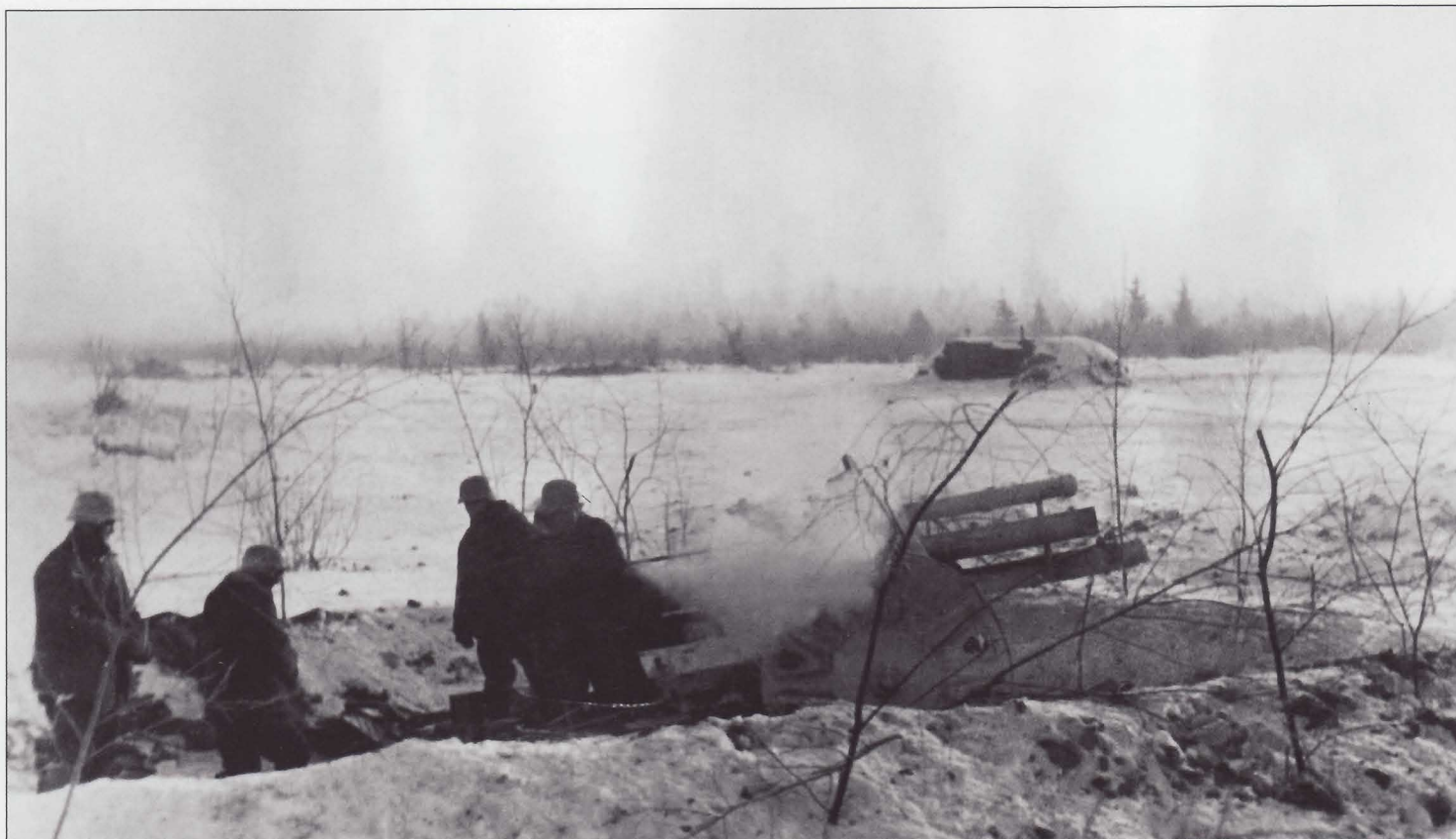
A 10.5cm I.F.H.18 light field howitzer (introduced in 1933) was the standard German divisional field artillery piece. While a few cut saplings have been stuck in this position's parapet, it was extremely difficult to conceal the large weapons in the winter. Besides muzzle flash and smoke, the muzzle blast kicked up snow. Moreover, white snow forward of the muzzle was scorched black or blown clear to reveal bare ground.
