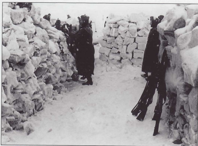
This frosty trench system is revetted with rocks. Coupled with many feet of frozen snow this provides a great deal of protection. In the spring thaw the snow will melt and portions of the stone facing will collapse. The position will have to be constantly reconstructed by repositioning rocks and adding sandbags and logs. The position might even be moved in the process because with the snow gone the lie of the land changes and positions can be shifted to more favorable terrain.
