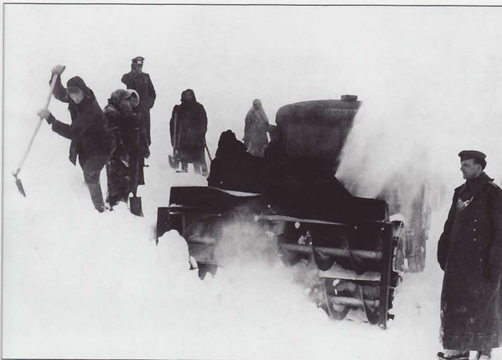
The Heer formed a number of different types of snow removal units (Schneeräumeinheiten) to operate snowplows and snow-blowers. It was critical that lines-of-communication be kept open for truck, wagon, and foot traffic. These units, under the pioneers (Pioniere), also kept airfield runways open. Here a snow-blower half-platoon (Schneefräsen-Halbzug) clears a road. These units were often augmented by Russian prisoners of war or local civilians, which explains the presence of a field military policeman (Feldgendarm) to the right.
