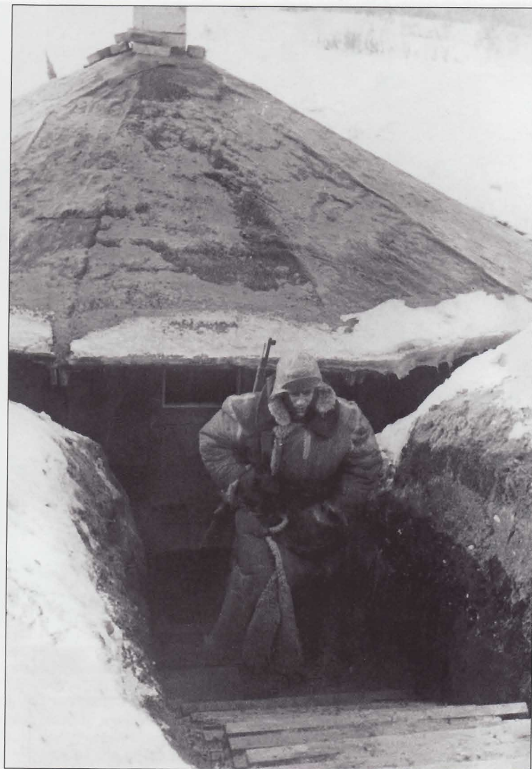
This frosty trench system is revetted with rocks. Coupled with many feet of frozen snow this provides a great deal of protection. In the spring thaw the snow will melt and portions of the stone facing will collapse. The position will have to be constantly reconstructed by repositioning rocks and adding sandbags and logs. The position might even be moved in the process because with the snow gone the lie of the land changes and positions can be shifted to more favorable terrain.
