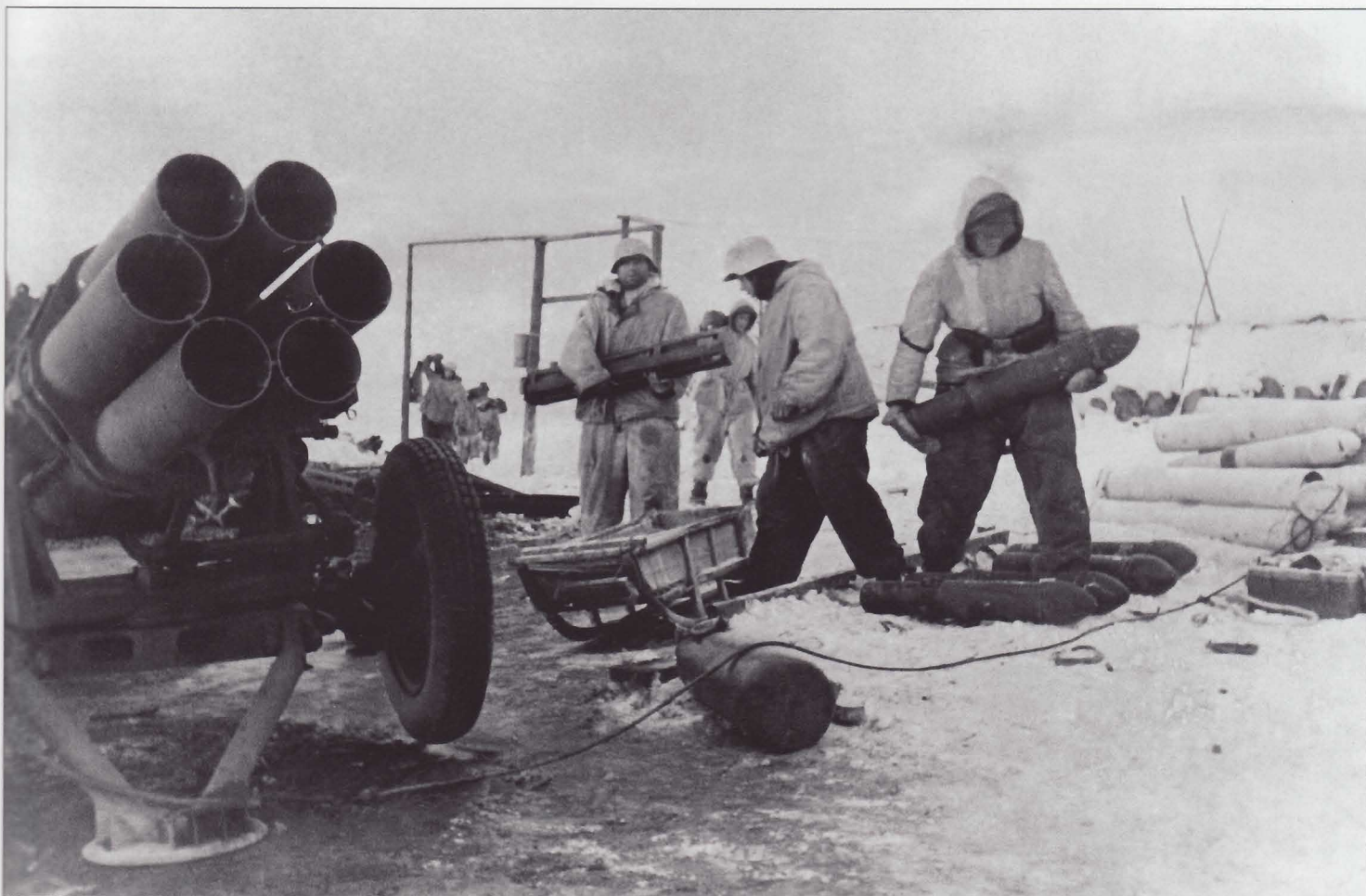
The crew of a 15cm Nebelwerfer 41 rocket launcher. The extreme cold adversely affected the performance of the high-explosive rockets, which were painted black. They had to be protected from the cold and were brought out into the open just before firing. The frozen solid propellant might fail to ignite or caused erratic flight path and widely varied range. The inaccuracy this caused was compounded by the fact that snow somewhat muffled the otherwise substantial blast effect. There was not a great deal of fragmentation caused by these rockets as the bodies broke up in large pieces, but snow and frozen ground reduced secondary fragmentation from gravel and rocks.
