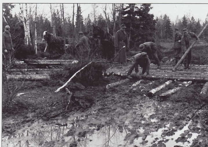
Pioneer troops lay a corduroy road through a marshy area. Only portions of roads really needing it were corduroyed owing to the amount of work necessary to fell, trim, move the trees to the road site, and emplace them. Five or six stringer logs were laid to support the road surface, more if the ground was extremely boggy. The road surface required a great number of six to eight-inch (150-200mm) diameter logs, nine to twelve per six feet (two meters). Then the chinks between logs had to be filled in with earth, gravel, bark, crushed twigs, etc. or the vibration would damage already road worn vehicles. Much additional effort went into maintaining corduroy roads as well.
