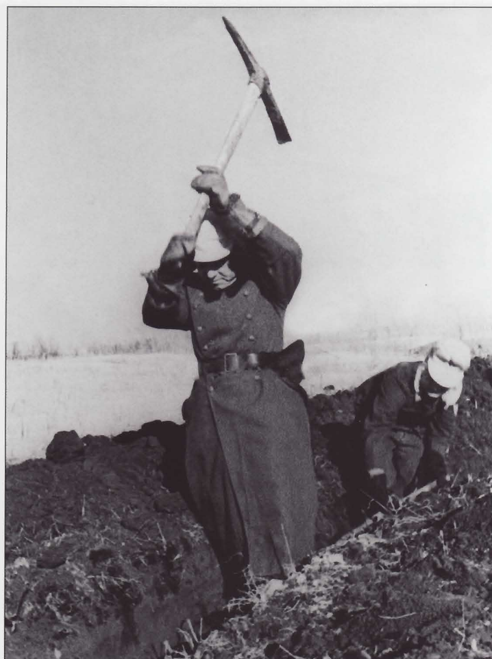
Digging a trench entailed a great deal of effort. The ground could be frozen solid from two to six feet (0.75 to 2 meters) depending on the duration of the freezing temperatures, amount of moisture in the spoil, thickness of snow and grass, and wind chill. Slit trenches were dug as narrow as possible, as little as 2 feet (60cm) for protection from aircraft strafing and artillery air bursts.
