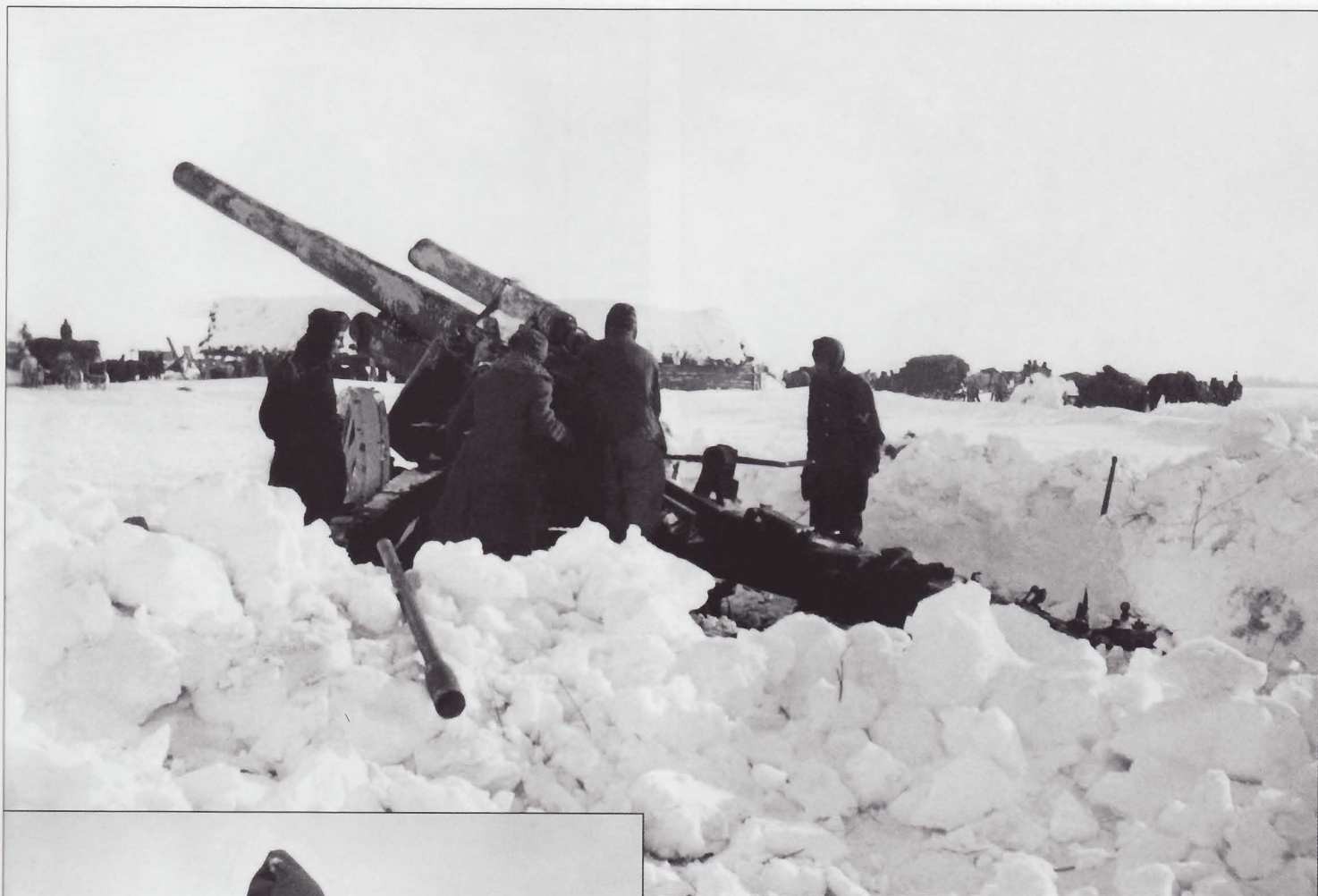
The Germans employed a number of different heavy non-divisional artillery pieces including this 15cm s.FH18 cannon (Kanone). This gun has been set up on level ground cleared of snow, which was piled as a parapet. It has been whitewashed in a splotchy pattern.
