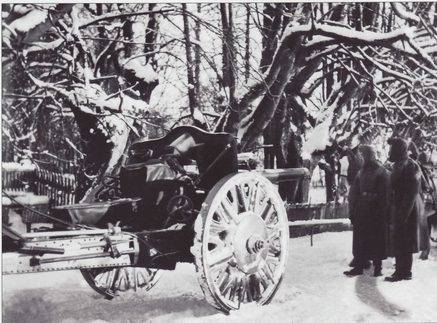
A 10.5cm I.F.H.18 light field howitzer attached to its limber. It could be towed by a team of six horses, a truck, or a 3-ton halftrack depending on the type of unit. Most were merely horse-drawn as here. The standard division had three battalions of these pieces organized into three four-gun batteries to total 36 howitzers.
