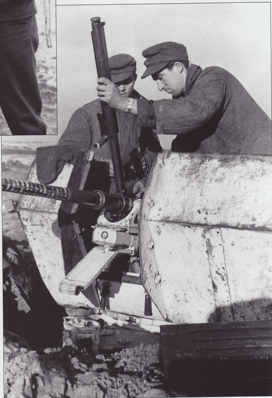
The crew of a 2cm Flak 30 remove the recoil cylinder for cleaning and adjustment. The gun shield and cradle have been whitewashed, but the gun itself was never painted.
