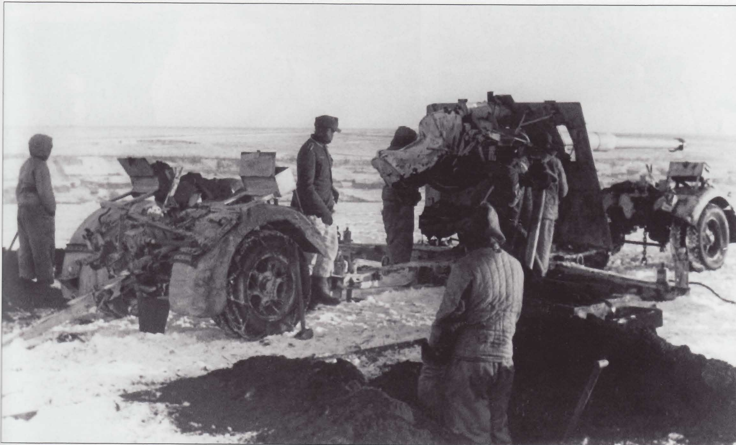
An 8.8cm Flak 36 is set up in a firing position on the steppes. The big gun was conspicuous and difficult to conceal much less dig in. The pit in the foreground is for ready ammunition. The "Acht-Acht" or "Otto-Otto", as the Germans called the "88", depended on its longer range to survive tank engagements. The ammunition handler standing in the pit wears a Soviet insulated winter jacket.
